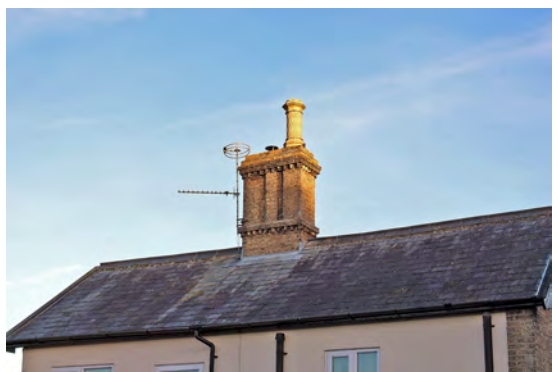
*18 A Victorian house slate roof
