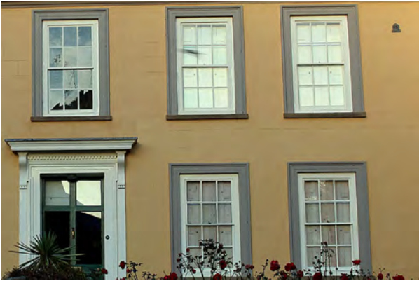
*3 Close-up of front elevation of Old Vicarage – wall panelling
