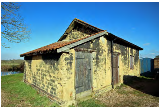
*9 Clay lump stable and small barn
