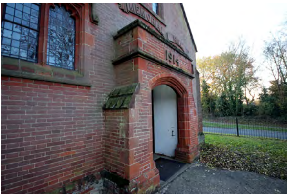
*7 Terracotta detail around porch entrance, Sancroft Hall
