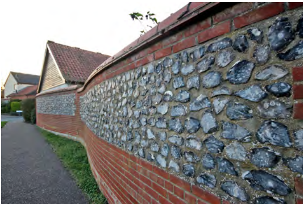
*5 Flint Walling at entrance to John Shepherd Road
