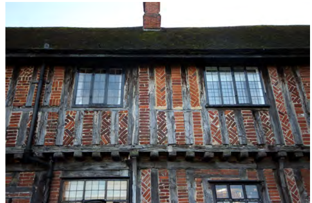
*6 Herringbone nogging work on Fox & Goose
