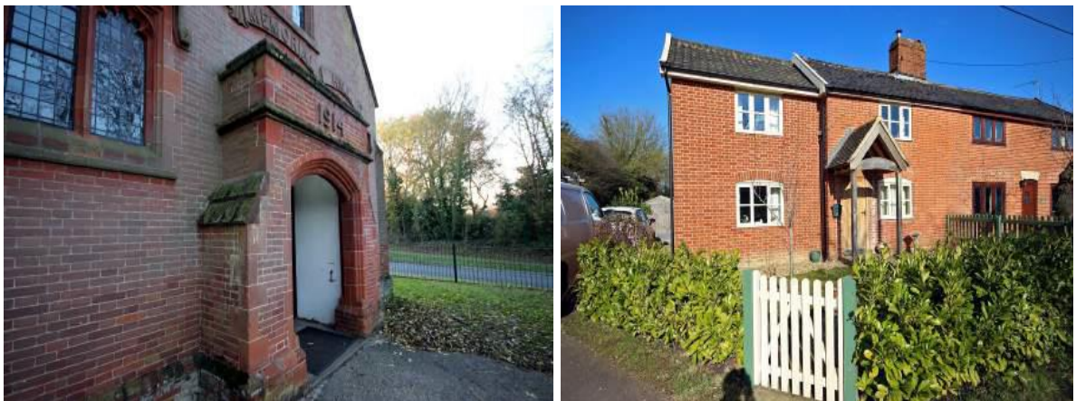
Details – porch details and brick arches
