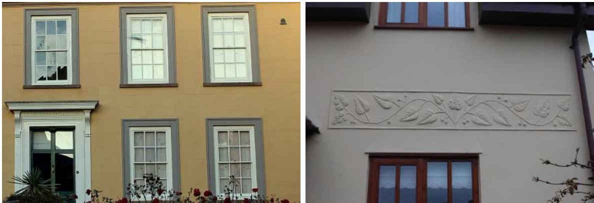
Details – wall panelling and pargetting
